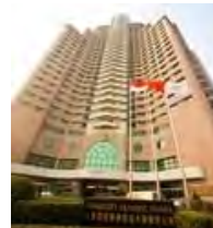
Somerset Olympic Tower Property Tianjin
